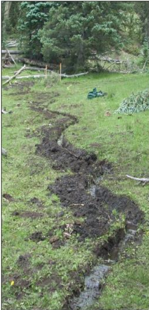
Figure 60. The photograph shows a worm ditch constructed by volunteers in the Springwagon Creek slope wetlands in the Comanche Creek Watershed. The schematic shows how to use a worm ditch in conjunction with other treatment structures to divert water out of an incised channel or gully.
